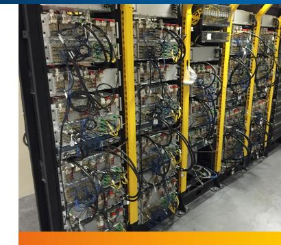
The Master Unit and sub-racks are **housed onsite** in the head-end room.
