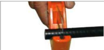
Straighten cable. Use RDCUTTER-S, applying even pressure around cable while rotating tool around cable to cut off cable squarely.
