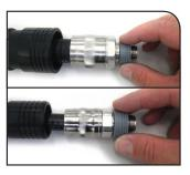
Prep the 1/2" cable and install the 1/2" connector. Refer to the JMA installation instructions. Install the port seal provided with the female connector.
